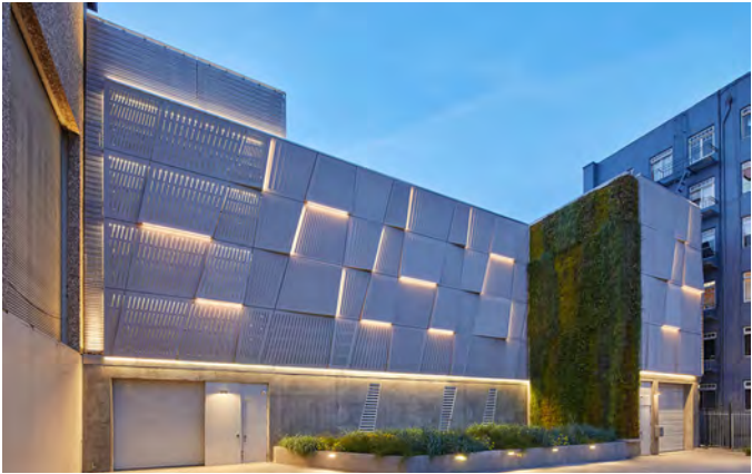
Larkin Switchgear Building – 2020 TEF Design AIA San Francisco, Architecture Merit Award, 2020 Architectural Record, November 2019
