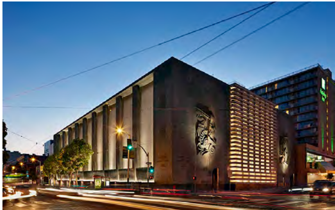
Mission Substation – 2014 TEF Design Published in Architectural Record, February 2016
