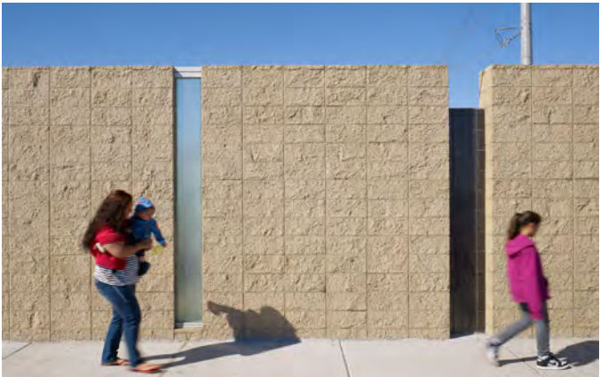
Martin Substation – 2014 TEF Design
