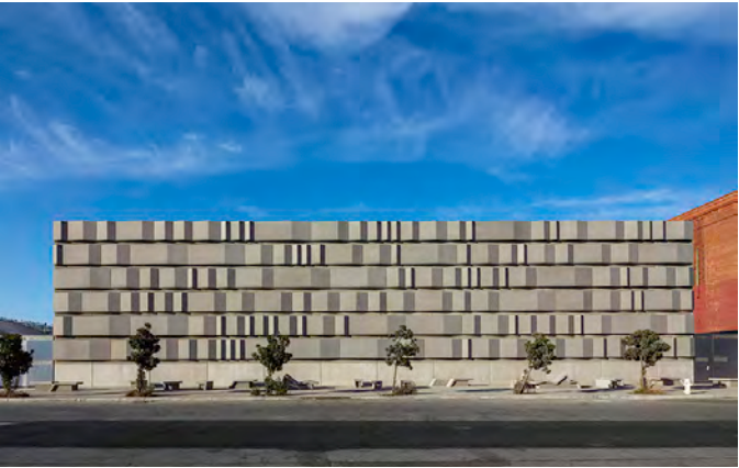
Potrero Substation – 2018 Stanley Saitowitz Natoma Architects AIA San Francisco, Architecture Citation Award, 2020 Architectural Record, August 2021
