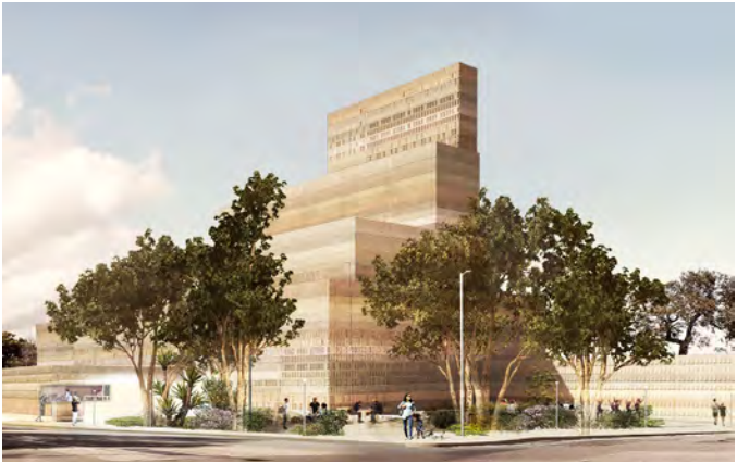
Hunters Point Substation 2016 – 2023 Tatiana Bilbao Estudio / TEF Design Advanced through pre-construction
