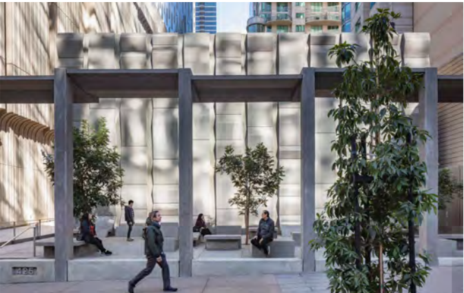
Embarcadero Substation – 2018 Stanley Saitowitz Natoma Architects Published in Architectural Record, August 2021
